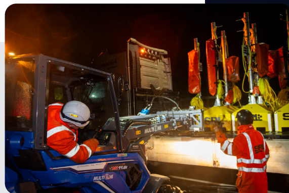
Above: Overnight installation with our experienced team.
